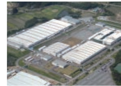
Soma No. 1 Aero-Engine Works
