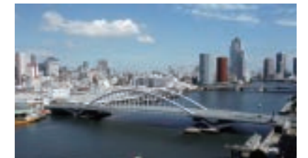
Arch bridge "Tsukiji Ohashi"
