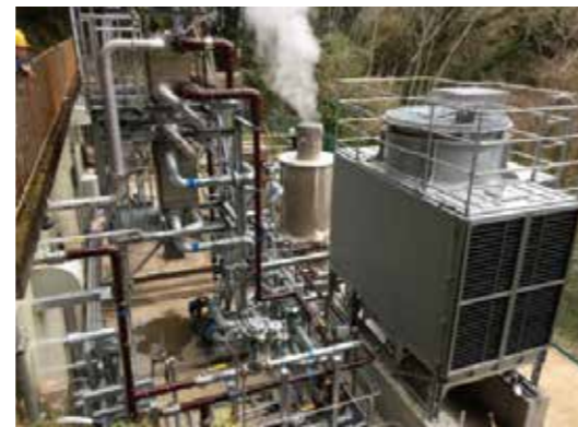
ORC power station using hot springs
