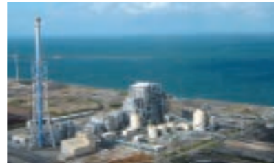
Boiler for IPP and PPS
