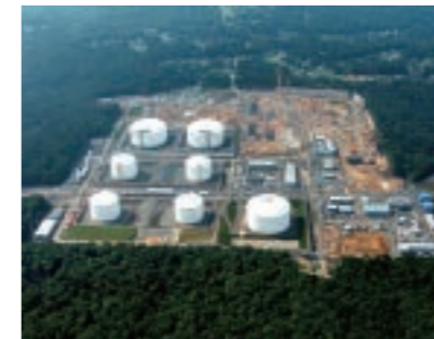
Natural Gas Liquefaction plants
