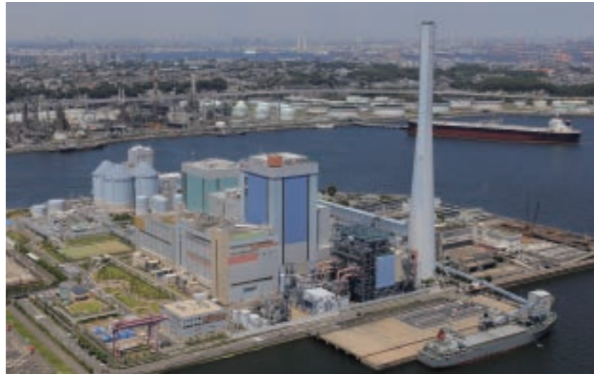
Large-scale tower type boiler Photo is provided by J-POWER (EPDC)
