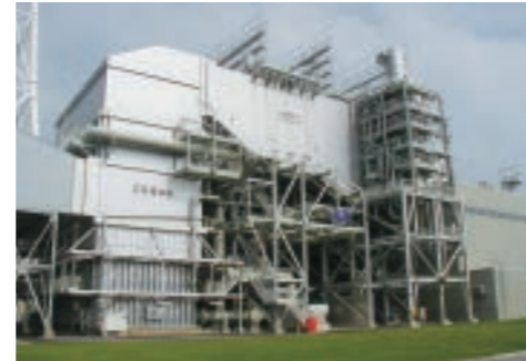
Flue gas treatment facility
