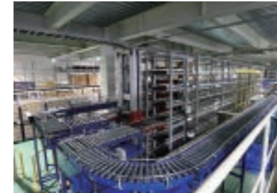
High-speed picking and storage system "Shuttle and Server"
