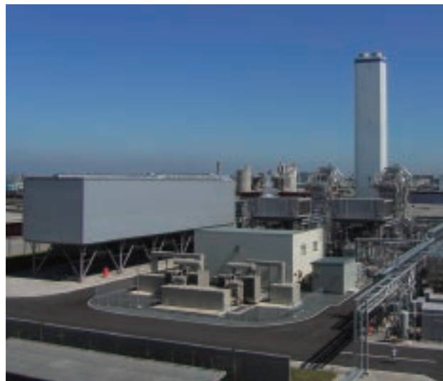
Gas turbine power plant "LM6000"
