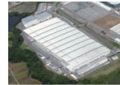
Soma No. 2 Aero-Engine Works
