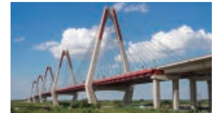
Cable-stayed bridge "Nhat Tan Bridge"
