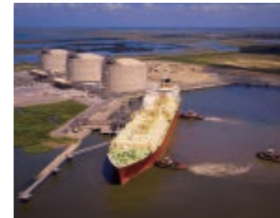
LNG受入基地 (Sempra向けCameron LNG受入基地(米国ルイジアナ州)) Photo used with the permission of Sempra LNG ©All rights received by Sempra LNG
