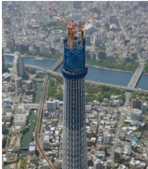
Jib climbing crane for building construction
