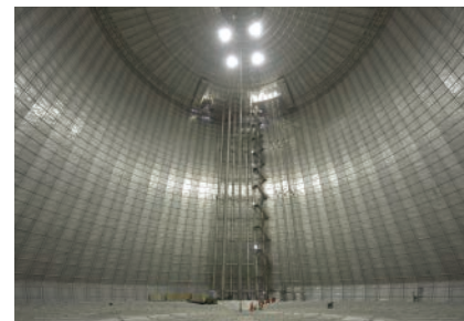
World's largest capacity LNG underground tank (Membrane) Photo is Provided by TOKYO GAS
