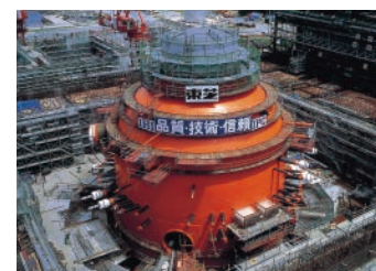
Reactor containment vessel
