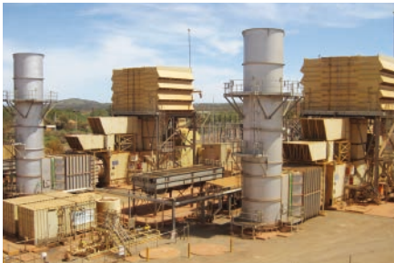
▲ Gas Turbine Power Plant (LM6000 Simple Cycle)
