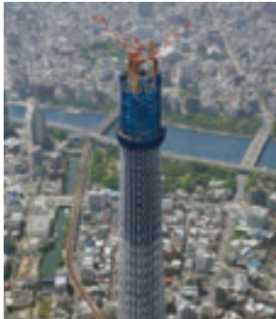
Jib climbing crane for building construction
