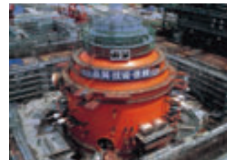
Reactor containment vessel
