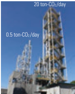
20 ton-CO 2 /day pilot plant for carbon dioxide capture and 0.5 ton-CO 2 /day demonstration unit at IHI's Aioi Works before shipment to Australia
