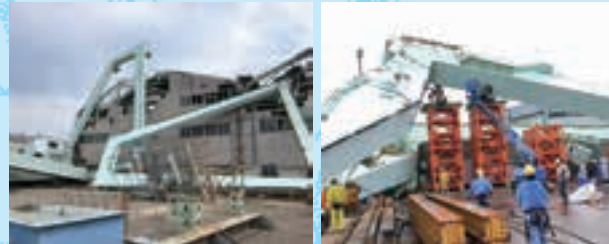
Cranes that collapsed at Sakai Works (left) and states of restoration (right)
