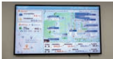
Monitoring of the energy management system control room
