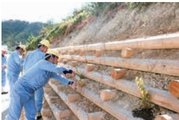
Planting activities at Aioi Works
