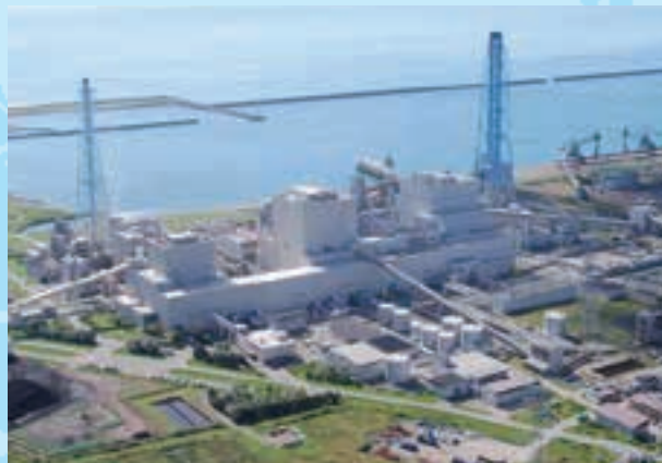
Tomato-Atsuma Power Station, Hokkaido Electric Power Company
