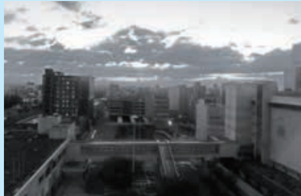
Tomakomai city during the power outage (4:37 am, September 6 th , 2018)
