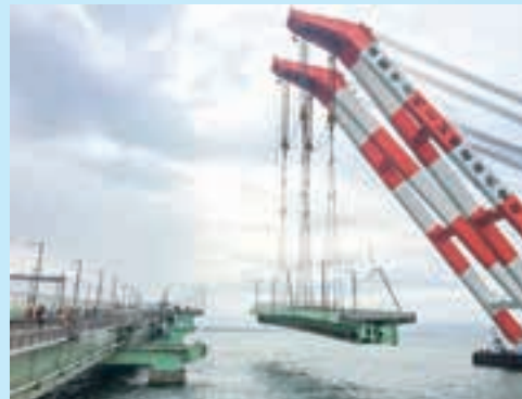
Removal status of damaged bridge girders
