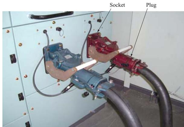
Fig. 5 AMP plug and socket on shore connection panel
