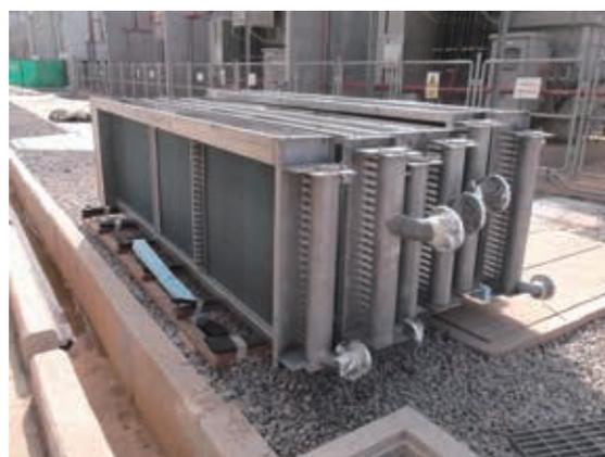
Inlet-air heating coil using steam
