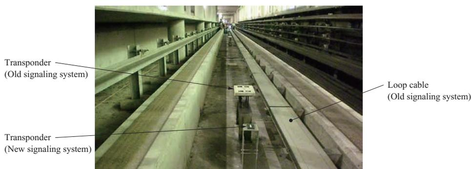
**Fig. 2** Trackside equipment for new and old signaling systems
