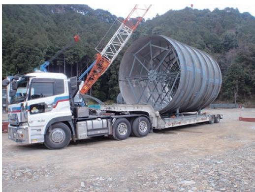
**Fig. 4** Transportation of the additional discharge pipe
