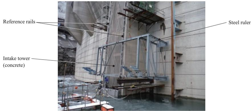
Fig. 9 Survey using the reference rail
