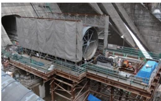
**Fig. 5** Coupling of the additional discharge pipes on the temporary steel stage
