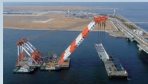
**Erection of large blocks using floating cranes**
