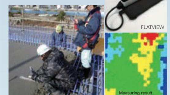
FLATVIEW can measure and visualize the flatness of the concrete surface before hardening. By measuring at the surface finishing stage, it is possible to instruct the plasterer as appropriate on the correction points, and it is expected that the correction work after the concrete is hardened will be reduced.
