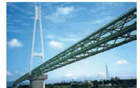
1995 Fukushima Prefecture, Niida Aqueduct Bridge (cable-stayed bridge type) (Pipe diameter: 500A x 2 rows, Span: 1198 x 2m)
