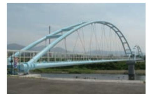
2008 Kagoshima Prefecture, Komenotsu Aqueduct Bridge (Basket-handle-shaped, Nielsen system Lohse type) (Pipe diameter: 300A, Span: 59.38 x 2m)
