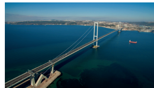
Osman Gazi Bridge (Turkey)
