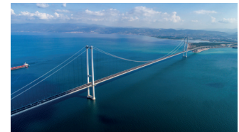
Osman Gazi Bridge, Turkey
