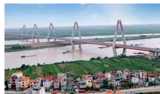
Nhat Tan Bridge, Vietnam
