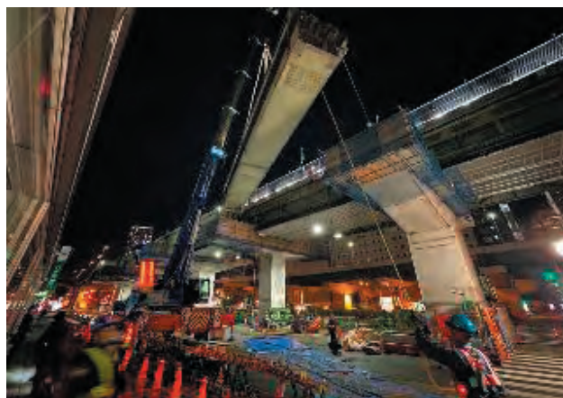
写真-5 既設拡幅桁撤去
