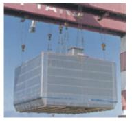
An SPB tank during installation on an LNG carrier
