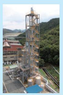
Chemical absorption method pilot plant
