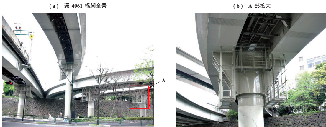
第 8 図 環 4061：隅角補強 Fig. 8 Pier C4061 : Reinforcement at beam-to-column connection
