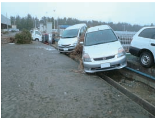
第3図 仙塩浄化センター震災直後（車の流出） Fig. 3 Photograph of the Senen Waste Water Treatment Plant immediately following the earthquake (cars swept away by the tsunami)
