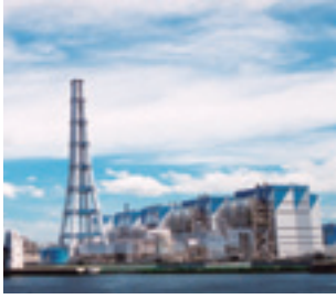
Boilers for power plants
