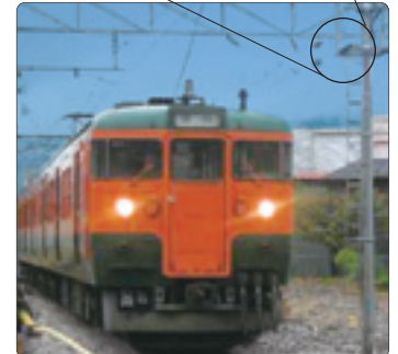
(Above) Obstacle detection system (Fig.1) (Below) 3D laser rader obstacle detection system installed in a railroad crossing (Fig.2)
