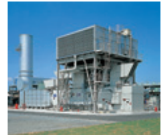
Gas turbine power plants
