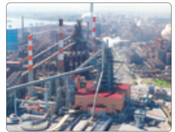
No. 1 Blast Furnace at Sumitomo Metal Industries' Kashima Steel Works
