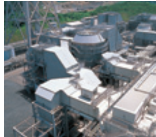
Air pollution prevention systems
