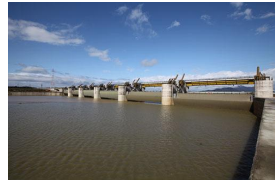
Okozu movable dam (completed Jan 2012)
