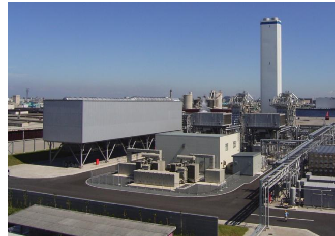
LM6000 gas turbine combined power generation facility
