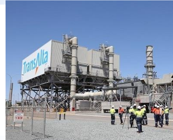
< "LM6000" power plant equipment >
