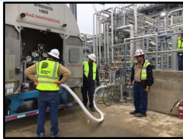
Liquid Ethane Unloading
