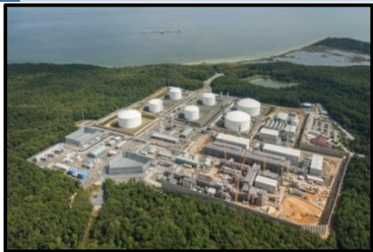
Aerial photo as of Sep. 2017
