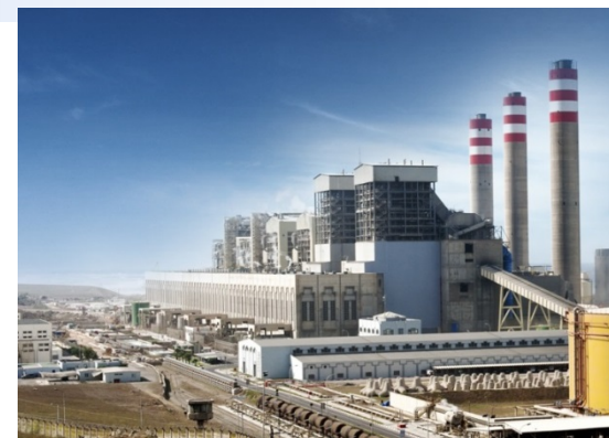
< Jorf Lasfar Power Plant >
