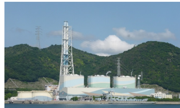
<Aoi Power Station>
