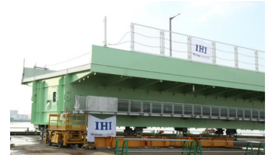
<Kansai International Airport Connecting Bridge, Outbound Line Girders>
