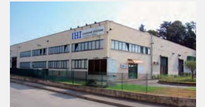
● IHI Charging Systems International S.p.A. (意大利)
