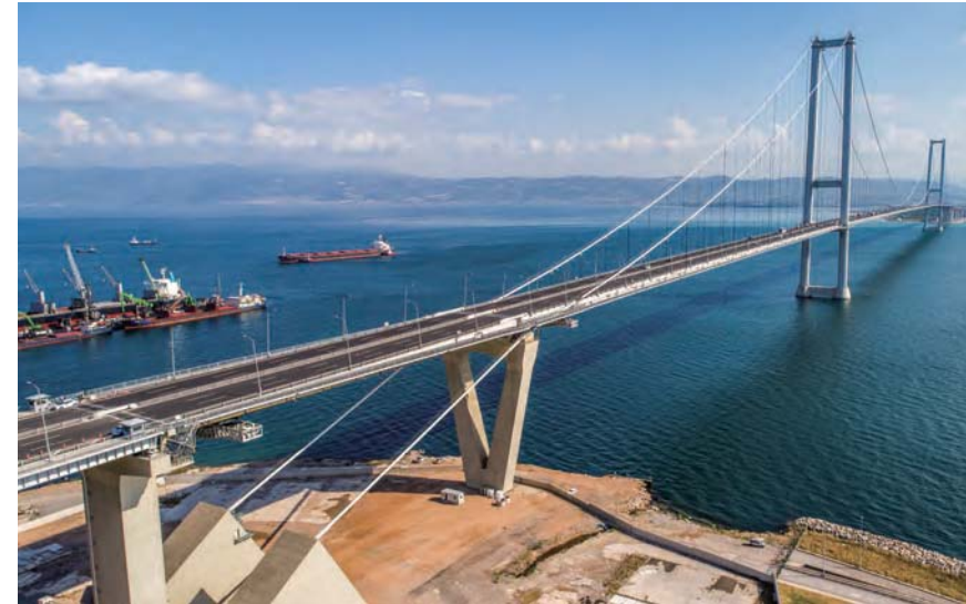
吊桥“Osman Gazi大桥”
