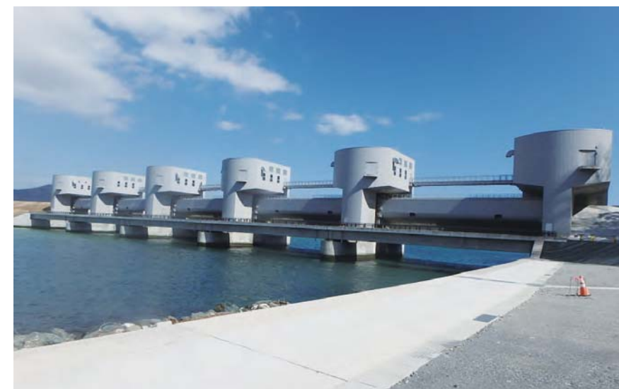
River gate (Kesengawa Gate)
