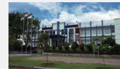
PT IHI POWER SERVICE INDONESIA (INDONESIA)
