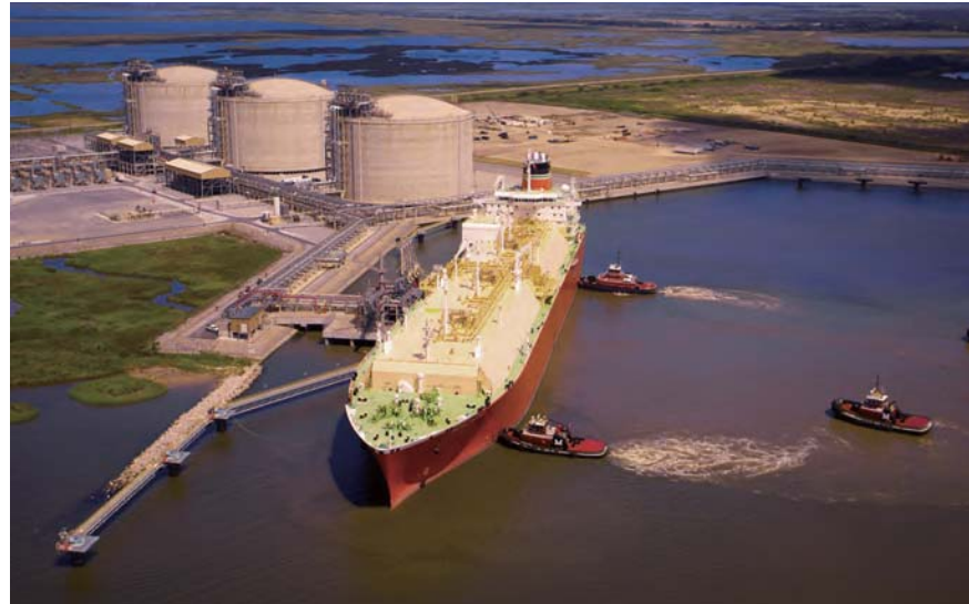
LNG receiving terminal (Sempra's Cameron LNG receiving terminal in Louisiana, USA) Photo courtesy of Sempra LNG ©All rights received by Sempra LNG
