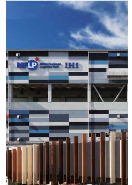
Mitsui Fudosan Logistics Park Toumei Ayase, which incorporates a medical evacuation heliport
