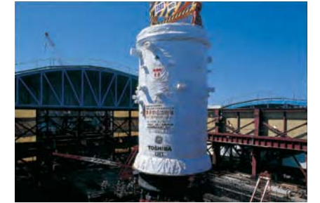
Reactor pressure vessel
