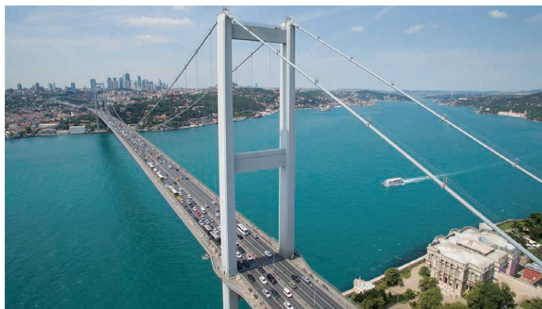
Fig. 9 Panoramic view of “Bosphorus Bridge”
