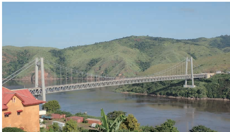
Fig. 14 Panoramic view of “Matadi Bridge”
