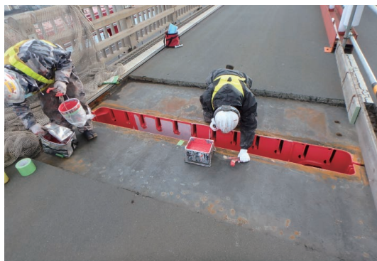
Fig. 7 Painting situation for joint of orthotropic steel deck
