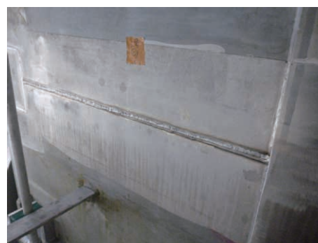
Passivation treatment at Tsuruda Dam
