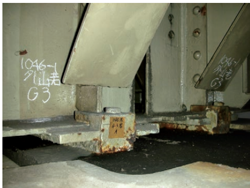
Fig. 13 Before and after replacement of bridge support
