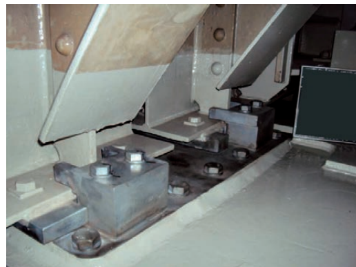
Fig. 13 Before and after replacement of bridge support
