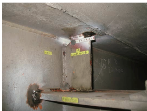
Fig. 25 Before and after replacement of web-gap plate
