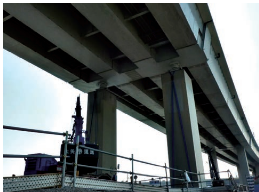
Fig. 32 Reconstruction of Bridge Pier 82 at Komatsugawa junction (6)
