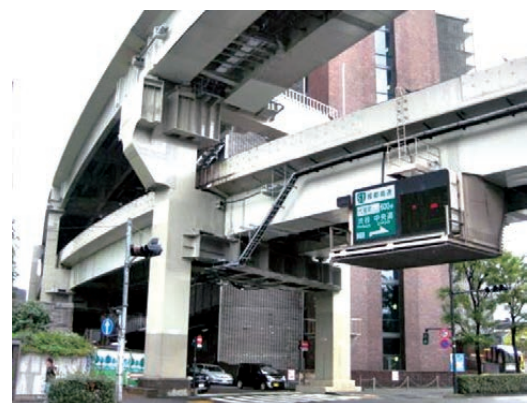
Fig. 7 Upper portion of Pier C4060 : Special support reinforcement
