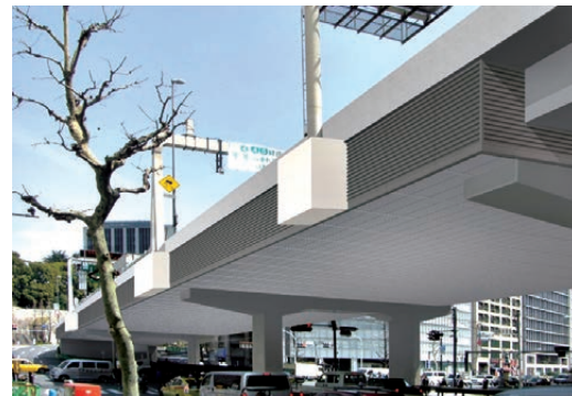
Fig. 34 New needs : Permanent scaffolding
