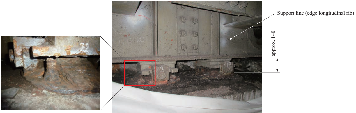
Fig. 27 Before replacement of bridge support (unit : mm)
