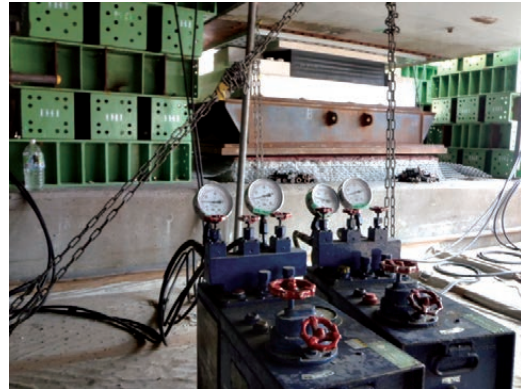
Fig. 16 Replacement of steel bridge support at intermediate support point
