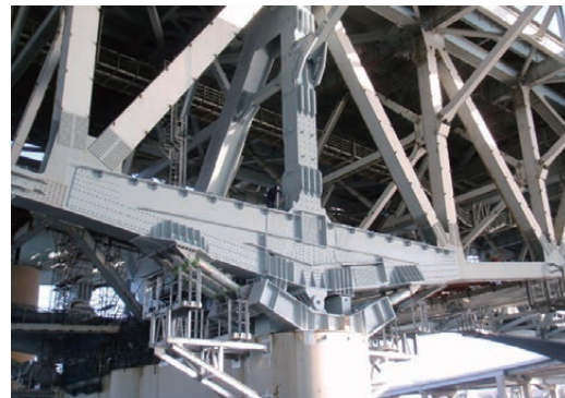
Fig. 20 Reinforcement at bridge support
