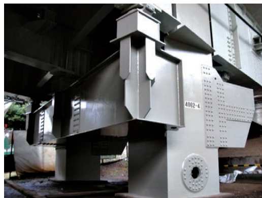
Fig. 9 Pier C4062 : Special reinforcing structure
