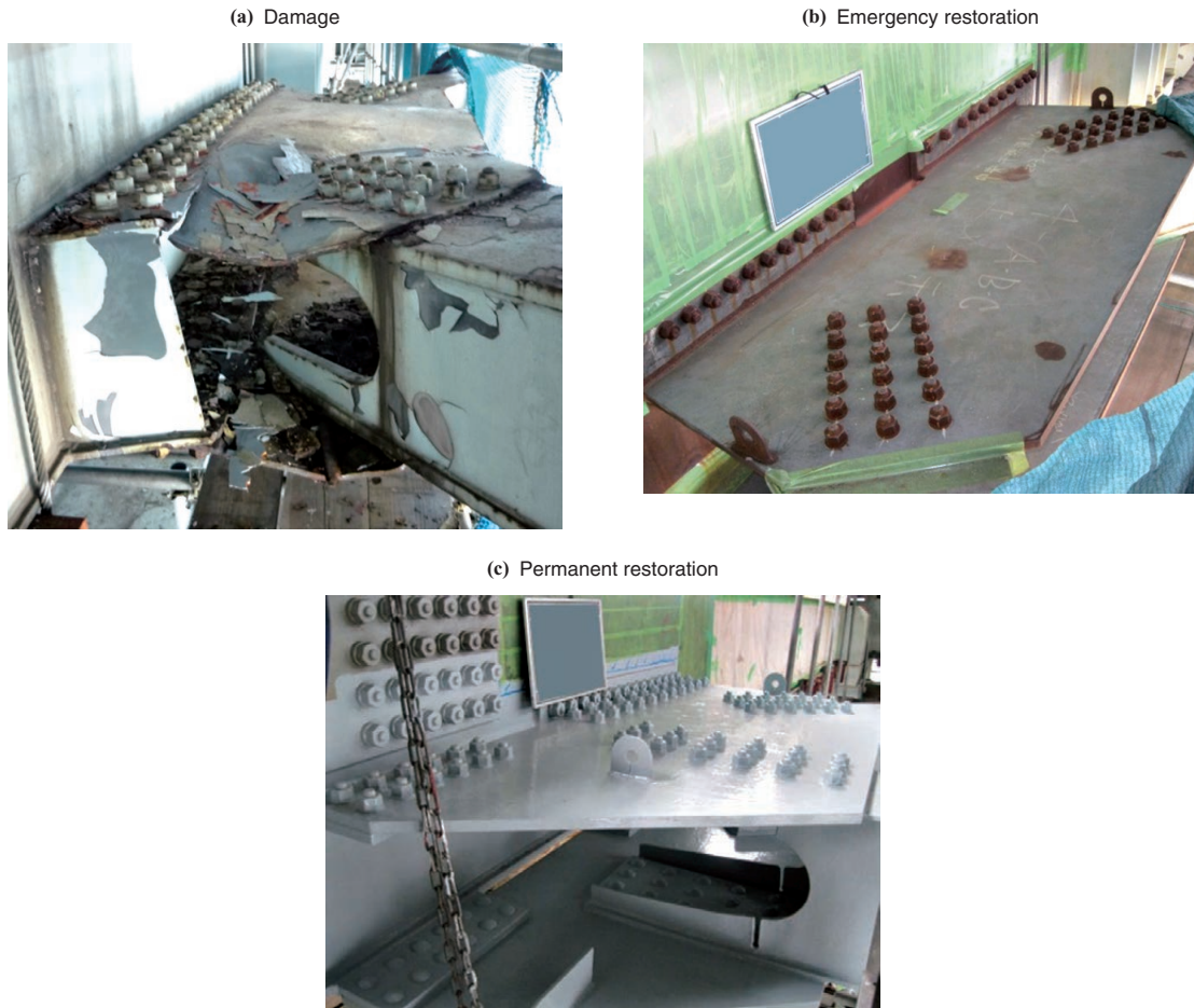
Fig. 21 Restoration of gusset plate
