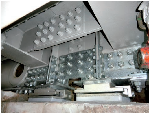
Fig. 28 After replacement of bridge support
