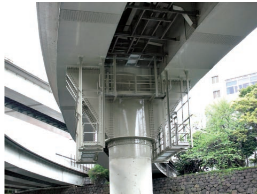
Fig. 8 Pier C4061 : Reinforcement at beam-to-column connection
