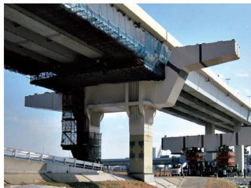
Fig. 32 Reconstruction of Bridge Pier 82 at Komatsugawa junction (6)
