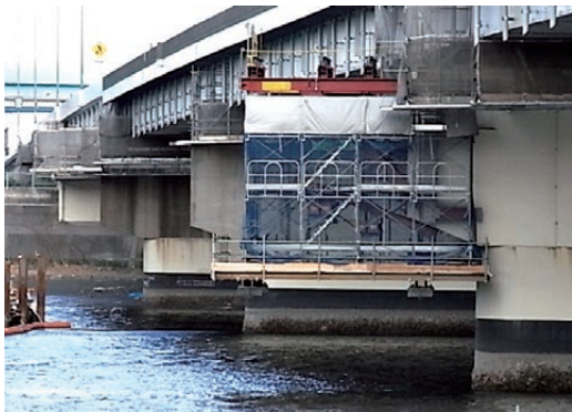
(a) Scaffolding erection
