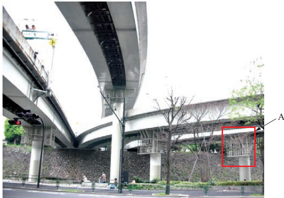
Fig. 8 Pier C4061 : Reinforcement at beam-to-column connection
