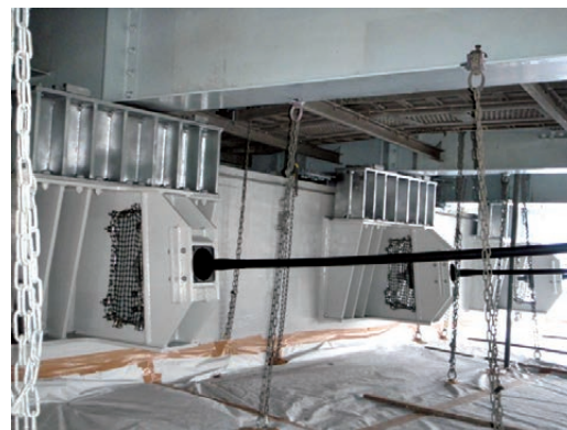
Fig. 15 Bridge collapse prevention and stepped prevention structure
