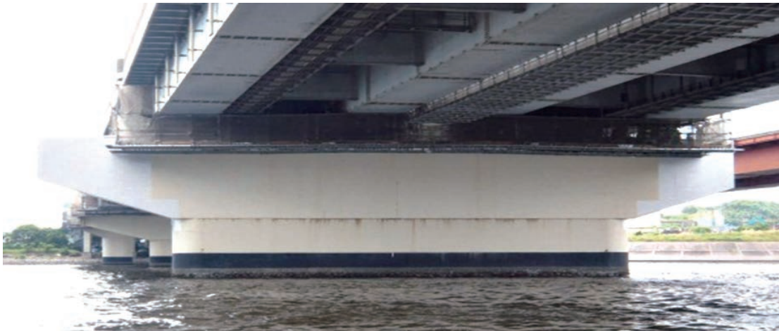
Fig. 17 Additional concrete beam at Pier B1516
