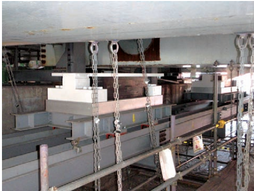
Fig. 16 Replacement of steel bridge support at intermediate support point
