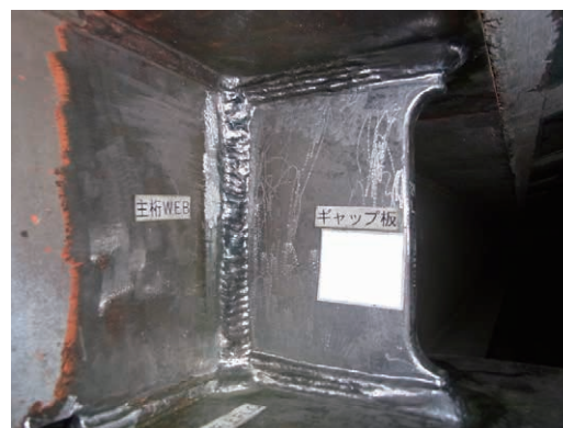
Fig. 25 Before and after replacement of web-gap plate
