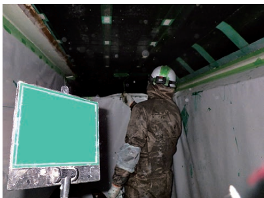
Fig. 30 Work status for carbon fiber reinforcement
