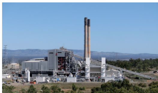
Callide Power Plant, Australia (30 MWe-class)
