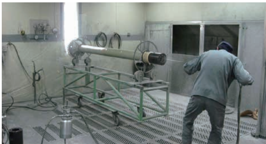
Coating work done by skilled worker
