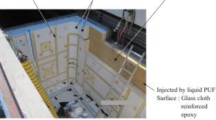
Fig. 6 Insulation panels and secondary barrier work
