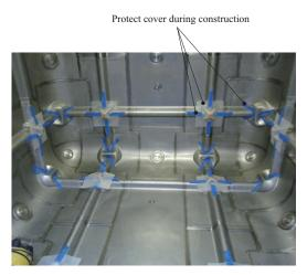
Fig. 10 Internal view of tank after welding of membrane
