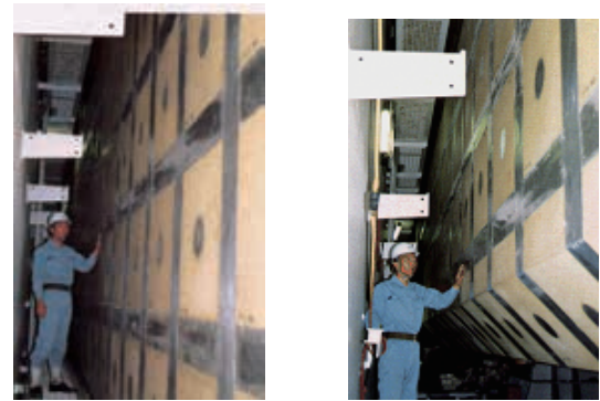
Fig. 8 Walkway between inner hull and tank outside insulation
