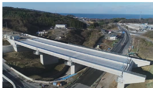
Fig. 25 Completion of construction of Taki PC upper bridge (2)
