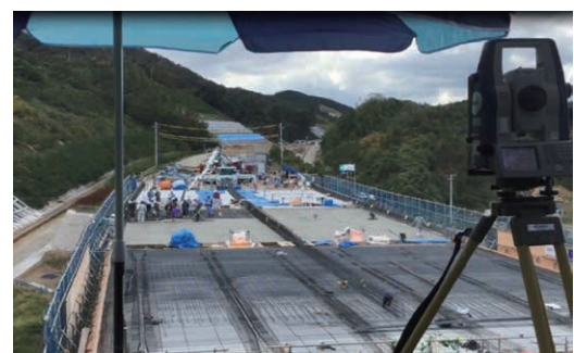
Fig. 16 Floor slab quality control using TS (2), (3)
