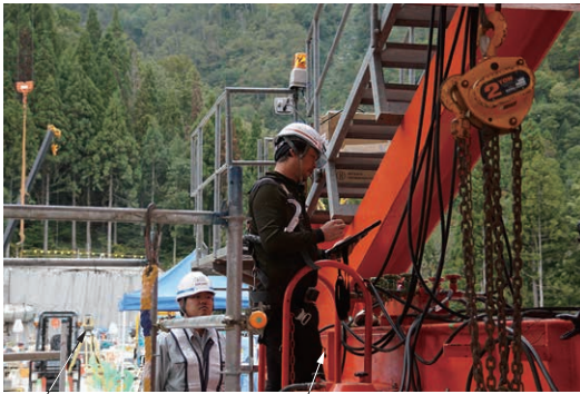
(a) Install a position information acquisition device
