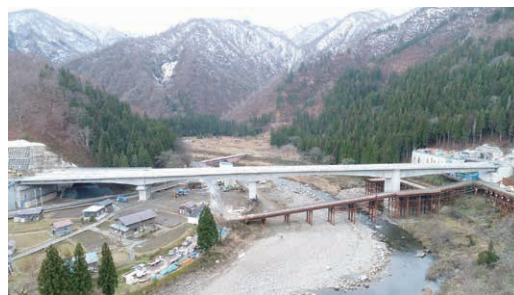
Fig. 26 Completed bridge superstructure of Kuzuryu River Bridge (2)
