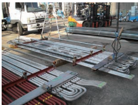
The 700°C-class verification test loop welded at the IHI Aioi Works
