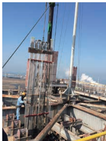
Installation of a 700°C-class verification test loop
