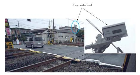
Fig. 6 Installation of 3-D laser radar level crossing obstacle detection system
