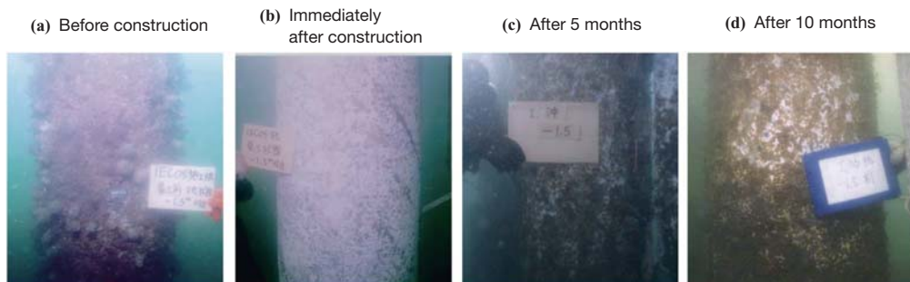
Fig. 14 Appearance of steel pipe pile surface
