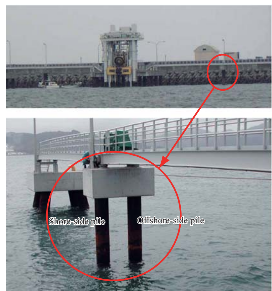
Fig. 12 Appearance of steel pipe piles under for marine tests
