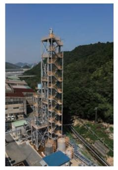
Chemical absorption pilot plant (20 ton-CO<sub>2</sub>/day)
