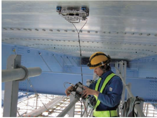
Fig. 11 Inspection under actual conditions from the bottom steel plate
