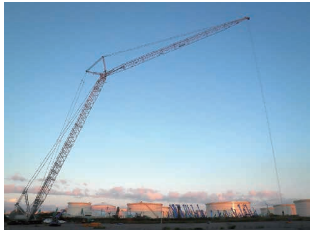
Fig. 1 Luffing jib crawler crane CCH3000LJ (Longest configuration)
