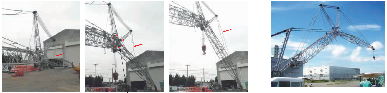
Driven mechanism for installing jib backstop
